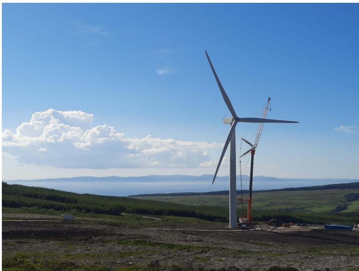
Diagram 4: Wind Turbine Erection at Blary Hill Wind Farm
