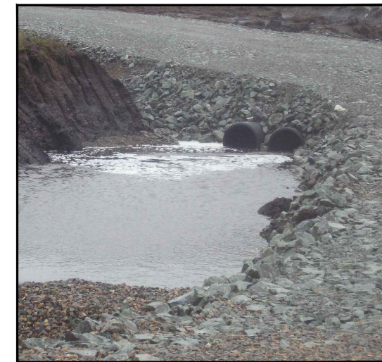
TYPICAL UNDER TRACK DRAINAGE
